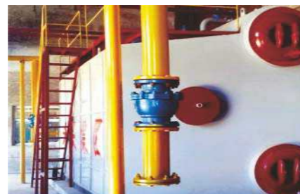
山西太原建筑企业 6吨过热蒸汽锅炉 6t/h gas superheated steam boiler for Shanxi construction enterprise
