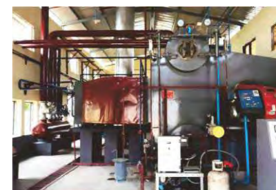
缅甸军工企业 15吨燃气蒸汽锅炉 15T gas steam boiler for Military enterprise
