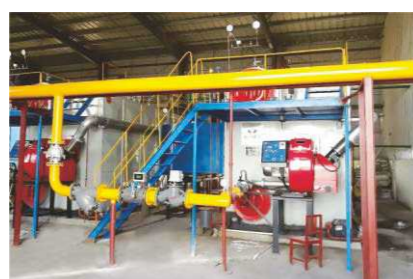
河南郸城薯业公司 10吨低氮冷凝锅炉 10t/h low nitrogen condensing boiler for Henan potato industry
